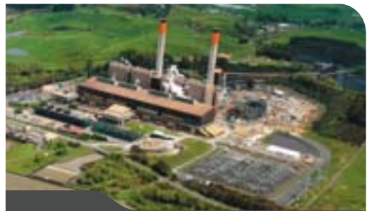
Cooling tower and e3p underway at Huntly
